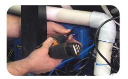
Re-attach the SpaNet™ controller panel.
